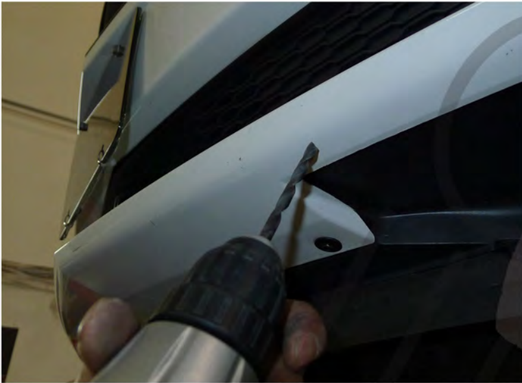
7. Drill with a .25 in drill bit
